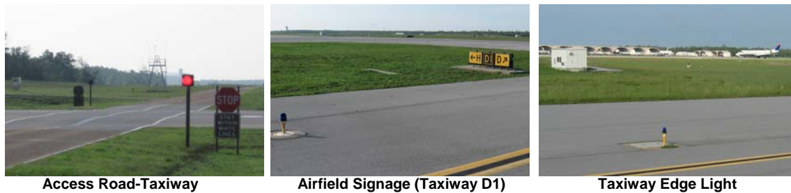
Figure 2-7. Airfield Lighting and Signage
